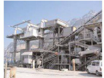
View of the grab dredge plant with parts of the transport system
