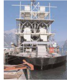
Front view of the two screening plants
