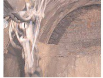
Terraced finish of the roof section.
